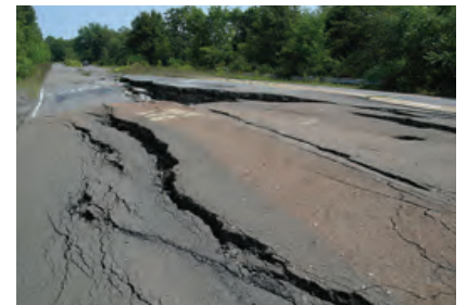
Infrastructure Ground Subsidence Issues
